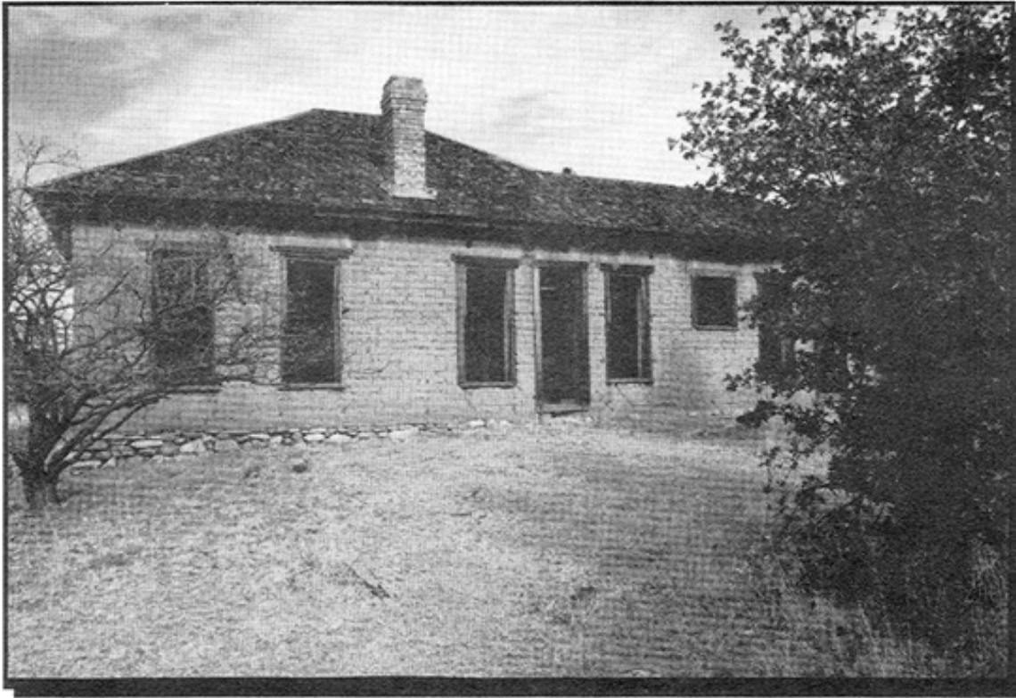
This adobe-brick building at southeastern Arizona's "Kentucky Camp" was originally the office of the Santa Rita Water & Mining Company. It was used later as a ranch house. This photo, courtesy of the Coronado National Forest office in Tucson, was taken in 1989 before the U.S. Forest Service began stabilization work.
